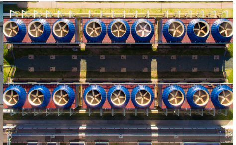
Chiller System Control
