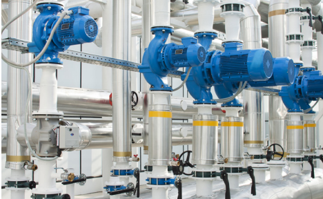
Water & Steam Boilers
