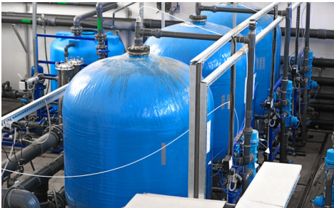
Wastewater Pump Control
